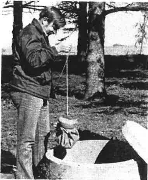
Fig. 2. Weighted sack filled with chlorine powder is lowered into the well.
